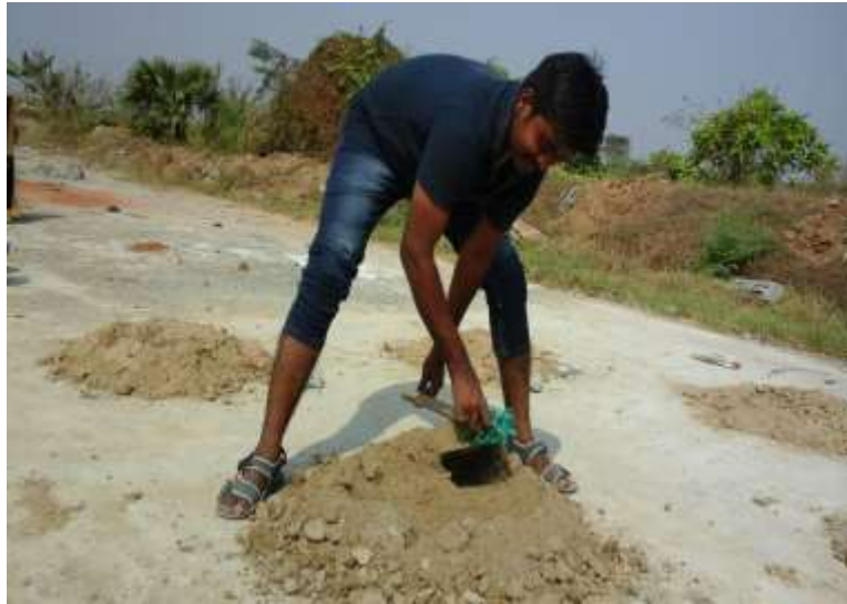
Figure 2.3 Mixing Of Materials
