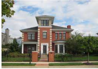
Figure 1.1 Construction using bricks
